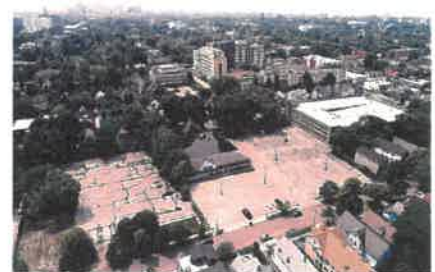
The site of the Elmwood Crossing development, which includes the former Women & Children's Hospital campus, the Gallagher parking ramp and a wide swath of paved area on Utica Street in the Elmwood Village. Buffalo News photo
